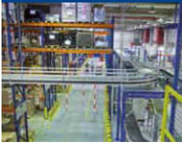
International Distribution Center
