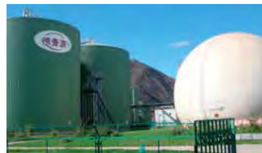
Biogas-digestors and storage tank
